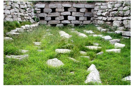
Remains of Ancient Linzi city sewer passing underneath the former city wall of the Qi kingdom.
